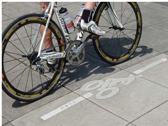
BICYCLE LOOP DETECTORS enable cyclists to trigger signals when vehicles are not present. Image Credit: NACTO
